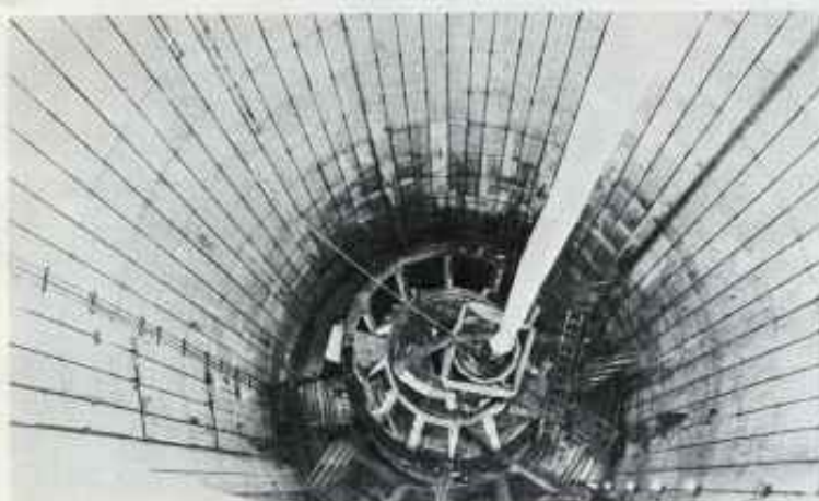
SPACE BOOSTER DIVISION'S gigantic cast-cure-test pit, 120 feet deep and 53 feet across, dwarfs a Minuteman first stage motor case undergoing propellant loading tests in Georgia. The pit has a 26-foot-thick reinforced concrete base.
