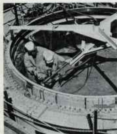
WASATCH technicians perform final machining operations on a segment case before propellant loading begins in a casting pit.
