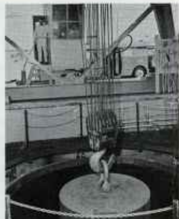
CYLINDRICAL mandrel, about the size of a Minuteman first stage, is positioned in a case prior to propellant casting.
